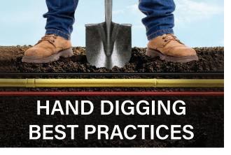
When your project requires you to dig within 2 feet of utility lines, mechanized equipment is not allowed. Hand dig to protect the underground utility line from damage.
