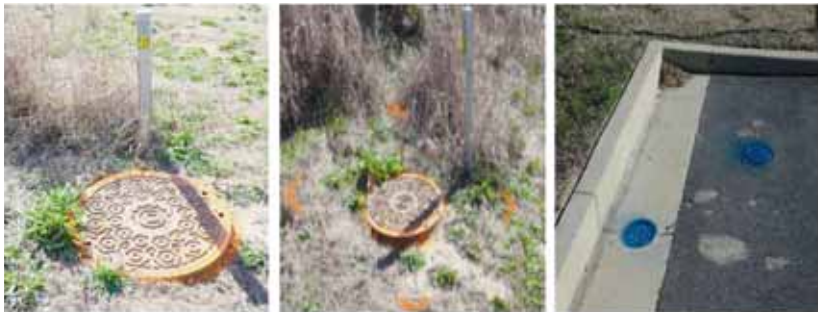
Manhole cover marking
