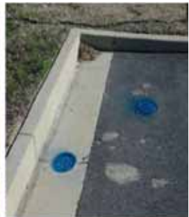
Valve box cover marking
