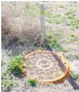
Manhole cover marking
