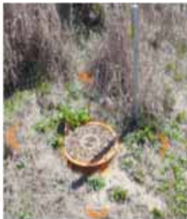
Manhole perimeter marking
